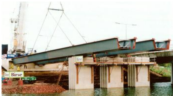
Figure 1: Open trapezoidal composite box girder during construction
