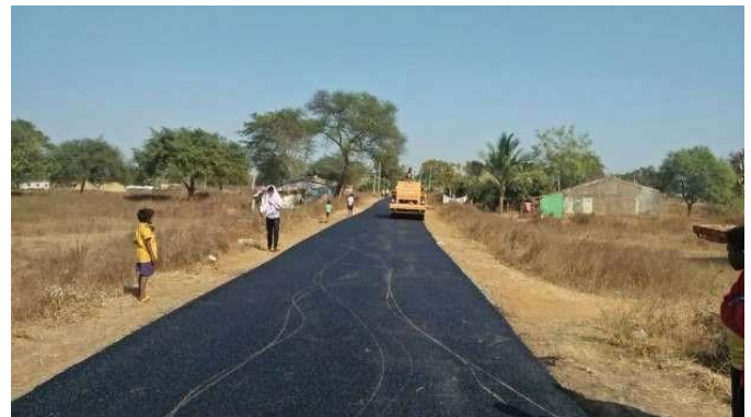
Fig 1.1 Construction of SDBC pavement
