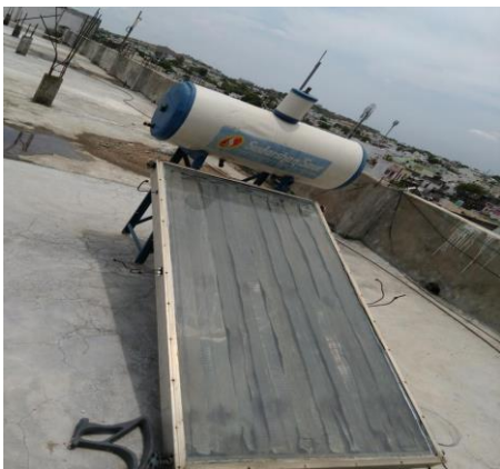
Fig. 4.1 : Solar Flat plate collector with straight riser tube
