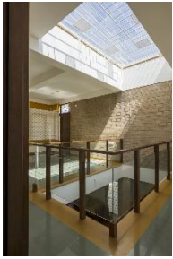
Figure. Skylight With Laser Cut Panels (Lcps)
