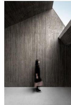
Figure. Showing anidolic zenithal opening
