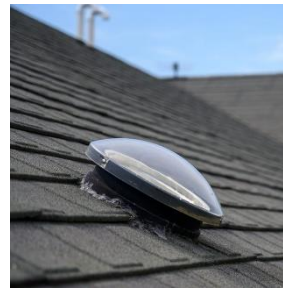
Figure. Solar Tube
