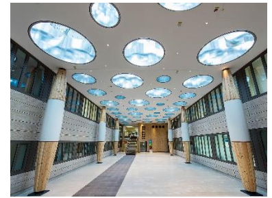
Figure. Light Pipe
