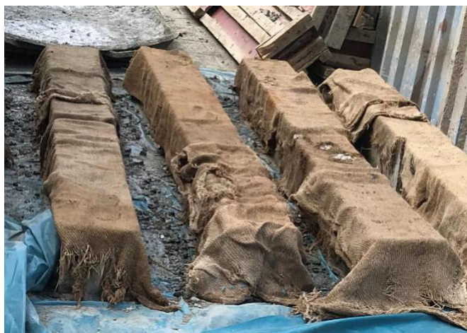
Fig No. 3 curing of concrete beam
