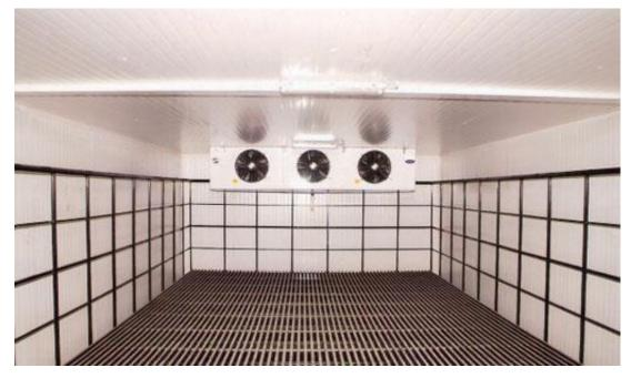
Fig.2 Evaporator located on the Top
