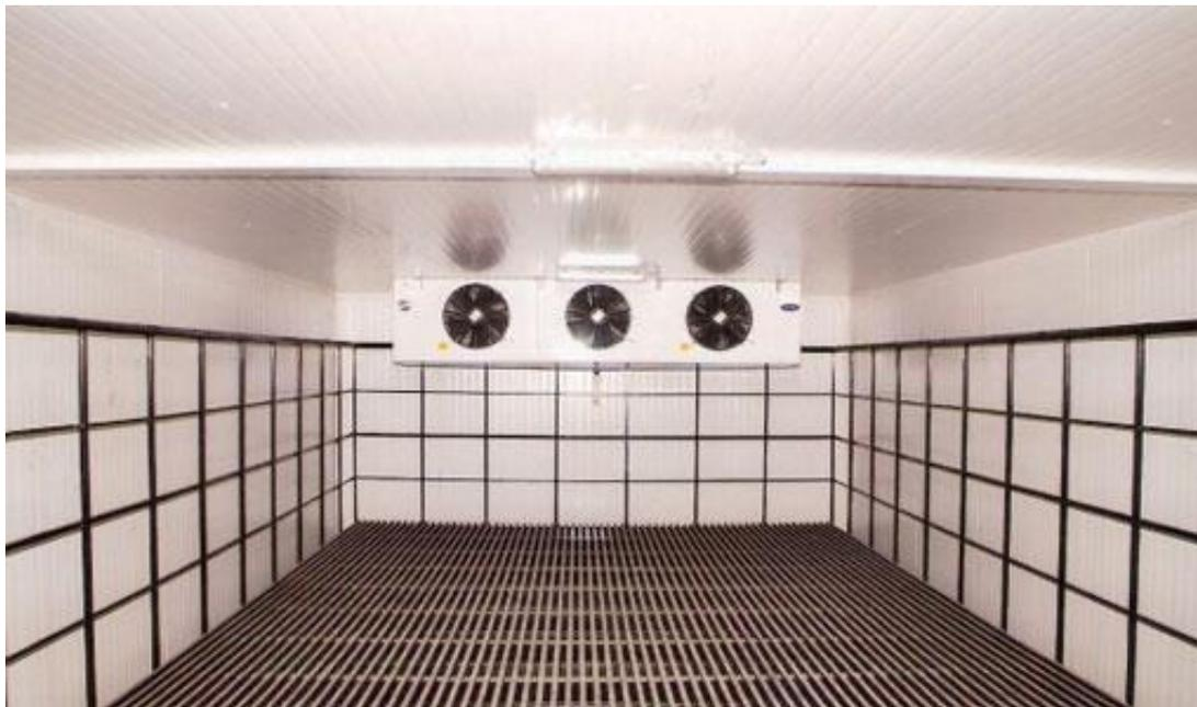
**Fig.2 Evaporator located on the Top**
