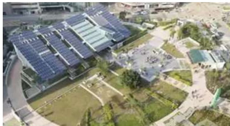
Figure 6: Onsite installed Solar PV Panels [20]
