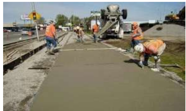
Fig 1. Road Grading construction
