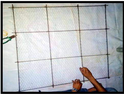
**Figure I: Tying of Reinforcement**
