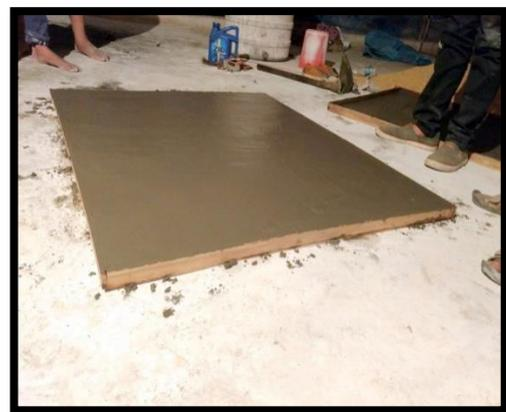
**Figure III : Casting of Slab Panel**
