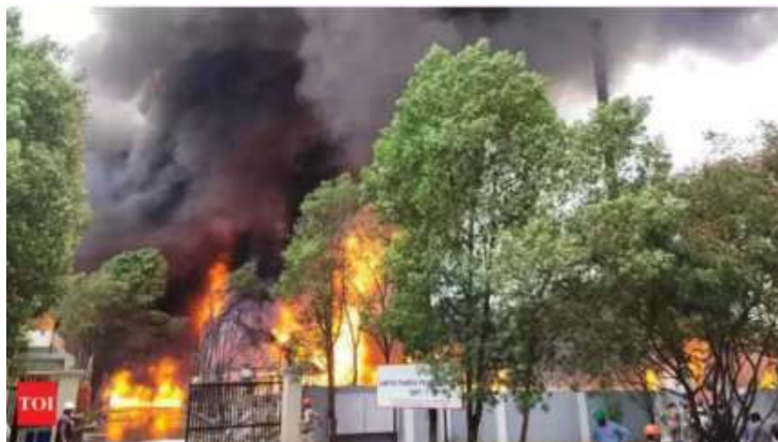
Figure 2. Atchutapuram Pharmaceutical Factory Explosion
