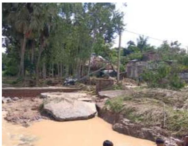
Plate No.3: Failure embankment near Billweswar
