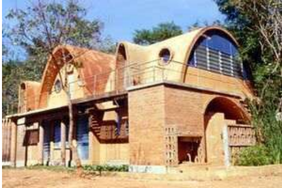
Fig -3: Auroville Earth Institute
