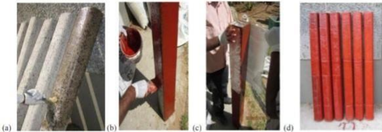
Fig. 4. (a) Application of Primer, (b) Application of saturant, (c) Application of GFRP sheet and (d) After application of GFRP sheet and saturant
