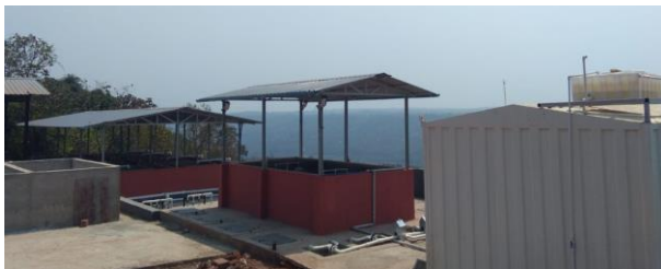
Overall Plant View
