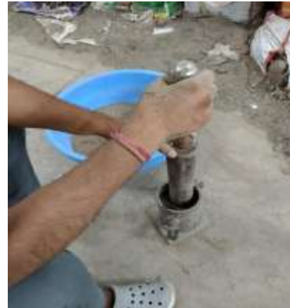
Figure 1.3 Performing Light SPT test
