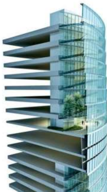
Figure 4: Double skin façade Shanghai Tower (Gensler Architects), Case study image in CTBUH database, 2018
