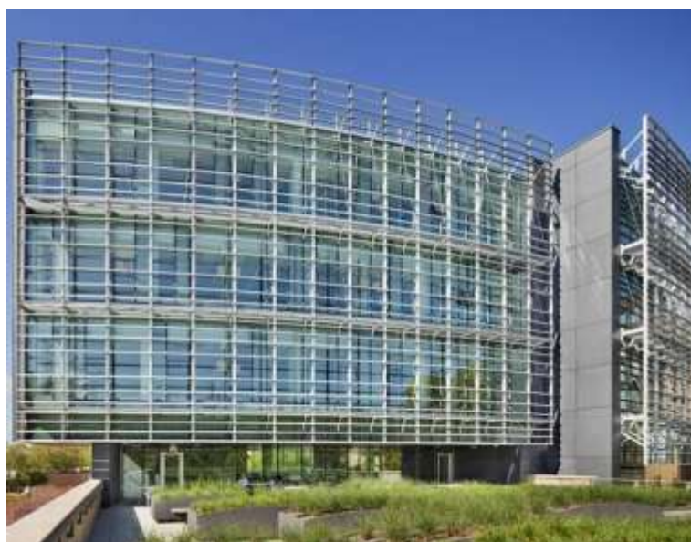
Figure 2: Motorised aluminium louvres for shading. Simon Centre for Geometry and Physics, U.S. (Architectural case study images, public domain).
