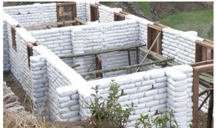
Fig 6: Earth Bag Walls
