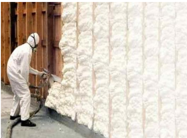
Fig 8: Polyurethane Foam Spray
