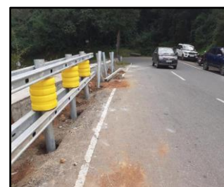
Fig-3: Installation of SRB at Ooty-Masinagudi Road
