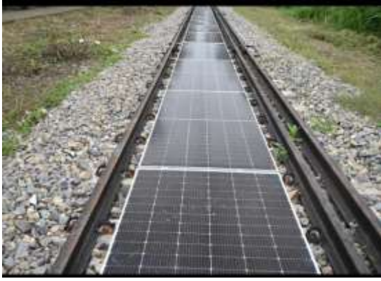
Figure(1) Solar panels on Railway tracks.
