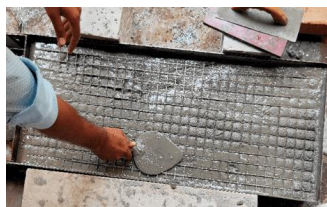
Top ferrocement layer
