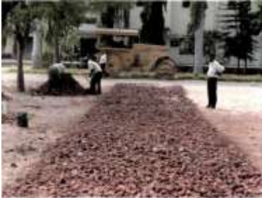
Fig. 1 Preparation of the aggregate layer below the slab.
