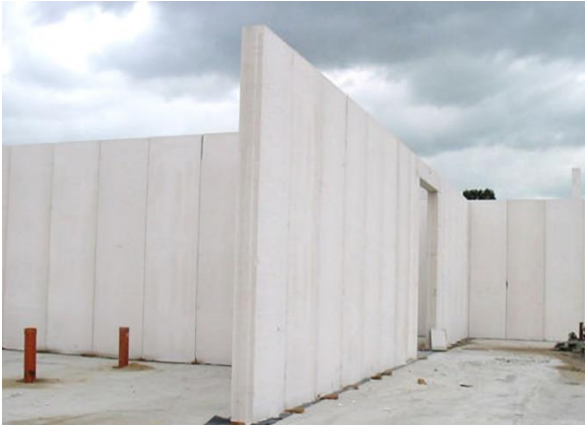
Fig 6 construction process of AAC panels
