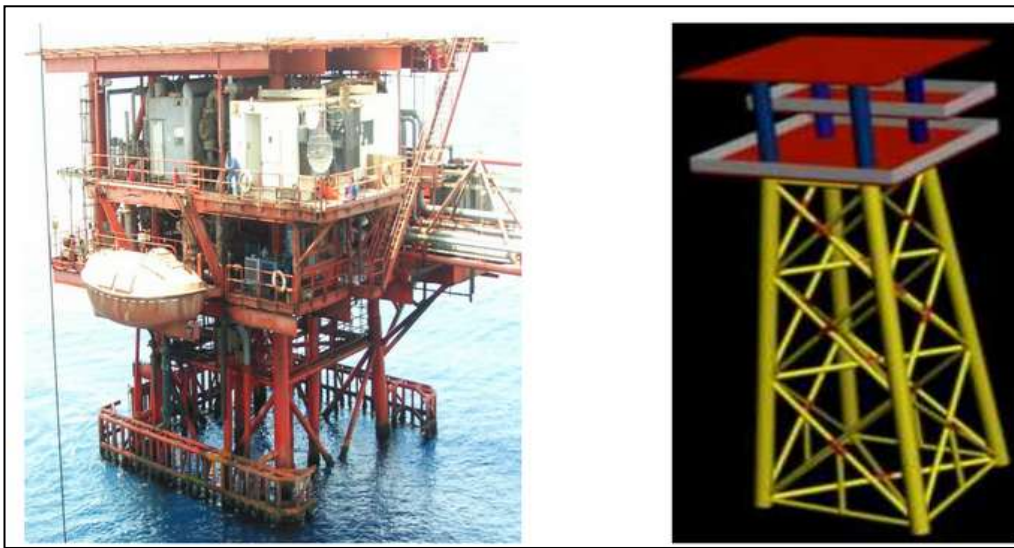
Figure 1. Typical Offshore Jacket Platform Model
