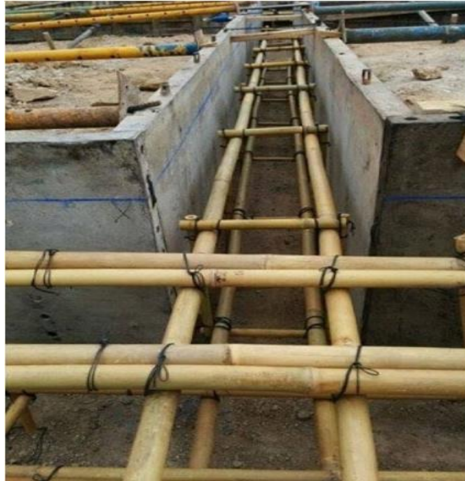
Fig. 3.1. Bamboo Reinforcement
