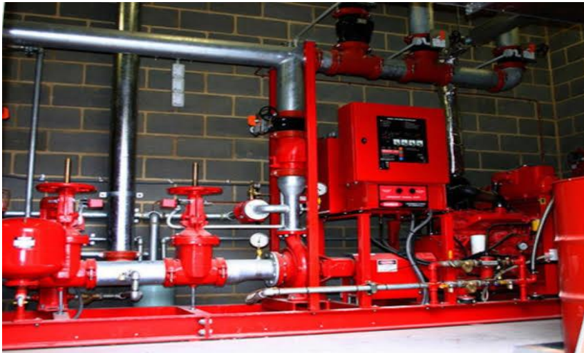
FIG 3.2.1 Deluge Valve OPERATION AREA
