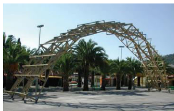
Figure 2 Mounted prototype of cylindrical folded structure formed by using wooden trusses as the elements of folded structure
