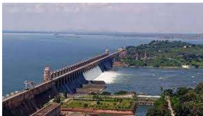
Fig -1: Overview of Tungabhadra Dam and reservoir
