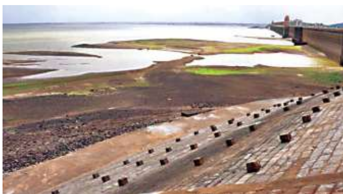
Fig -2: Tungabhadra reservoir at reduced water level exposing silt deposition
