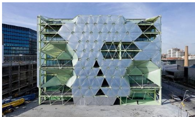
Fig. 6: Smart envelope comprised of ETFE encased solar-activated lamella shades developed for the Media-TIC building in Barcelona
