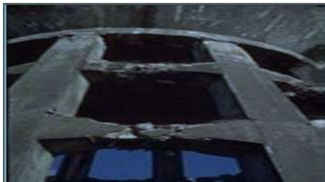
Fig. 1: RC Frame Staging of an Elevated Water Tank
