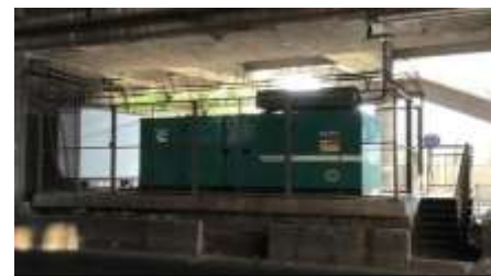
DG on road level under a Line 1 metro station
