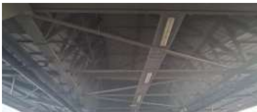
Nets to prevent pigeons from sitting on the roof of Ghatkopar Metro Station
