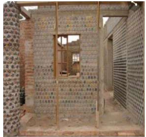
Fig 2. Plastic Bottle Constructed Wall
