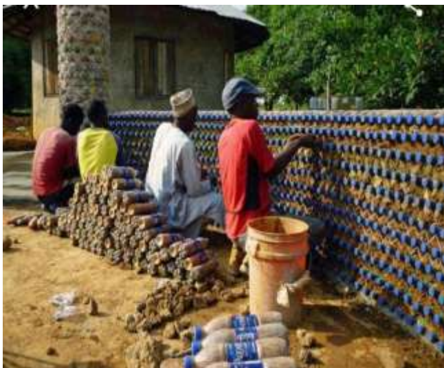
Fig 1. Plastic Bottle Construction
