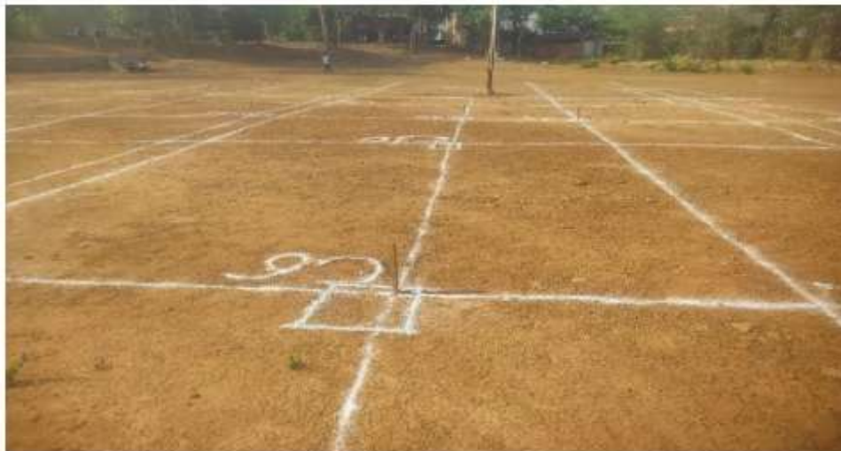
Fig. 14. Marking of Grid Lines
