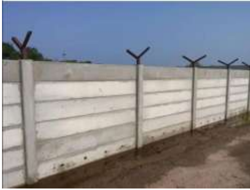
Fig -1: Crane-assisted erection of precast posts/panels
