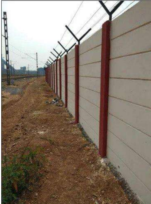
Fig -2: Completed boundary wall with security fittings
