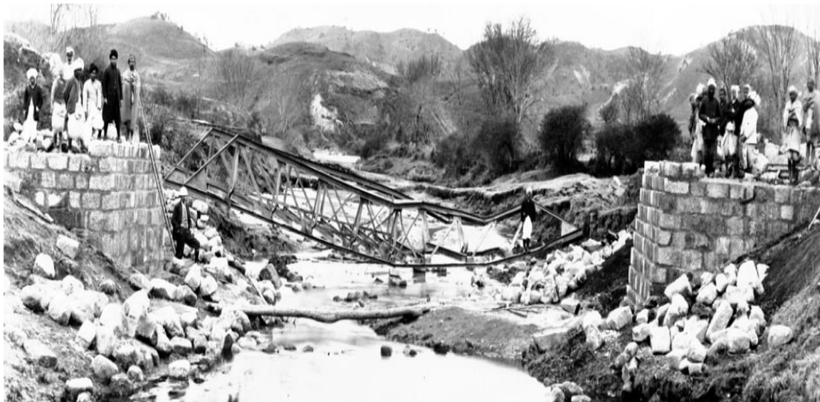
Figure 5. Shillong bridge toward Dawki: Impact of Earthquake 1897
