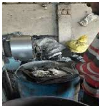
(B) Mixing of materials,
