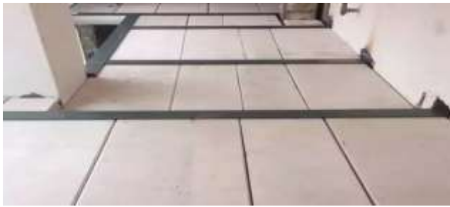
Fig. 4: AAC Panel Slab System
