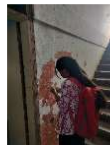
Fig. 2: Rebound Hammer NDT on RCC Columns
