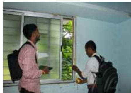
Fig. 1: Visual Inspection and Defect Documentation
