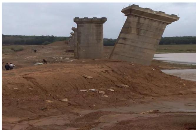
Fig no 1.1 settling pier
