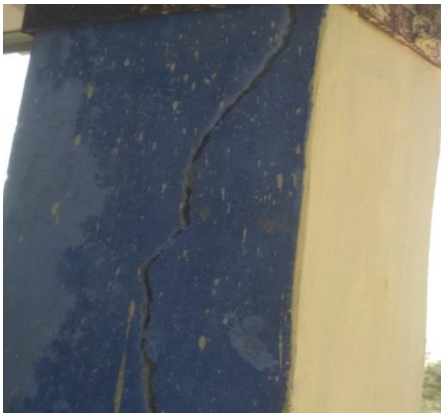
Fig no.5 Collapsing column (Source: Author)
