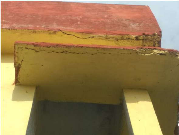
Fig no.3 Breakage in slab
