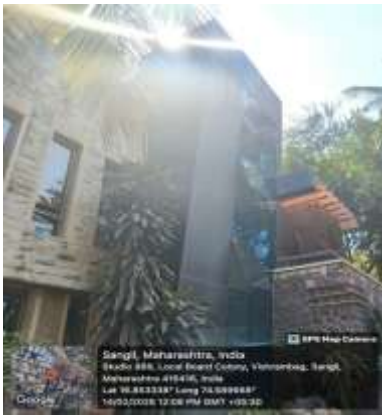
FIG 5- VACUUM WALLS AT STUDIO 888 IN SANGLI
