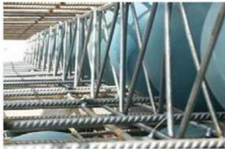
FIGURE 9: DIAGONAL GIRDERS STRUCTURE
