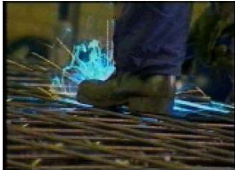
FIGURE 8: WELDING THE REINFORCEMENT
