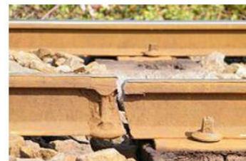
Fig. 1. Crack on track
