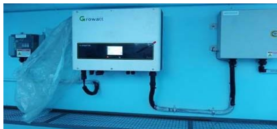
Fig. 5 Growatt Grid Connect Solar String Three Phase Inverter- 6 KW
