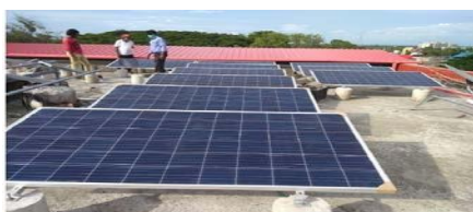
Fig. 4 Solar Modules, 325W/330Wp Multi crystalline
