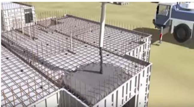
Fig.1. Monolithic Structure with Aluminum Formwork
