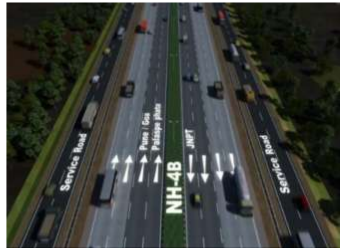
Fig -4: Revamping of existing road networks
