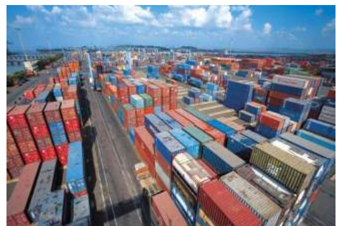
Fig -5: JNPT Port 4 th Container Terminal
