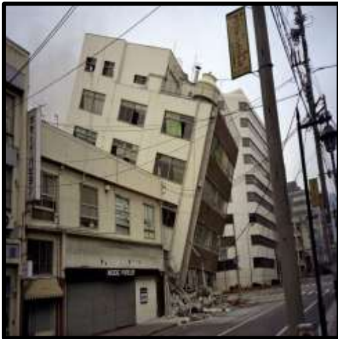
(e) Kobe Earthquake
