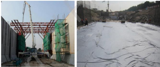
Figure 5. (a) Pouring of SHC (b) Curing of SHC (X. Zhang & Qian, 2020)
