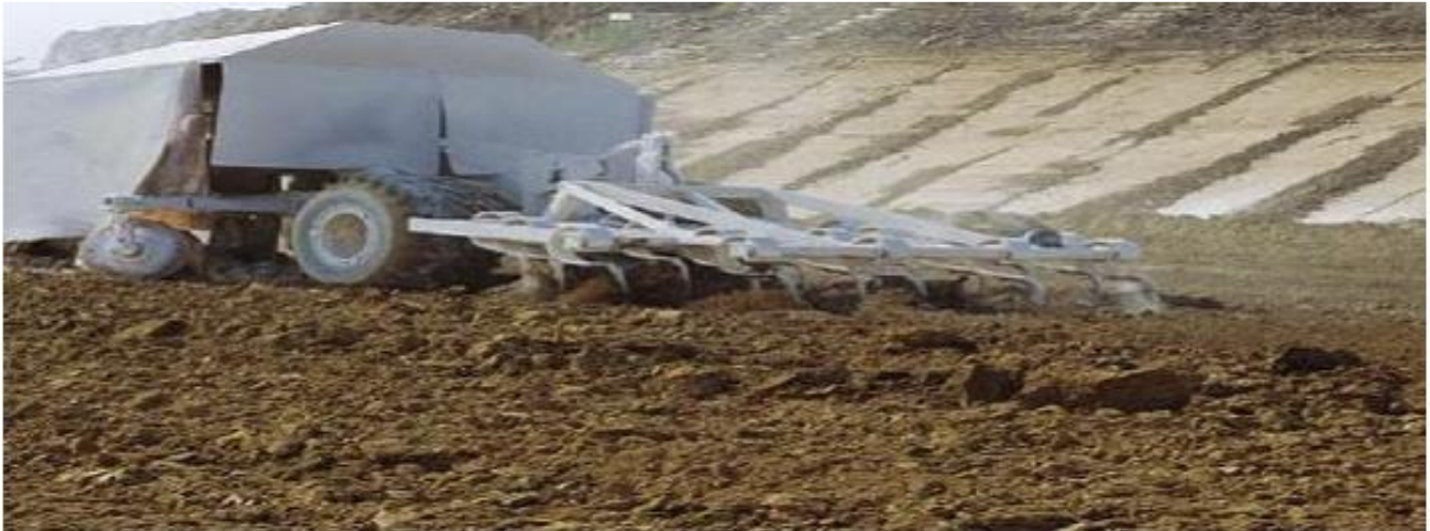
Fig. 2 Scarification before lime application
