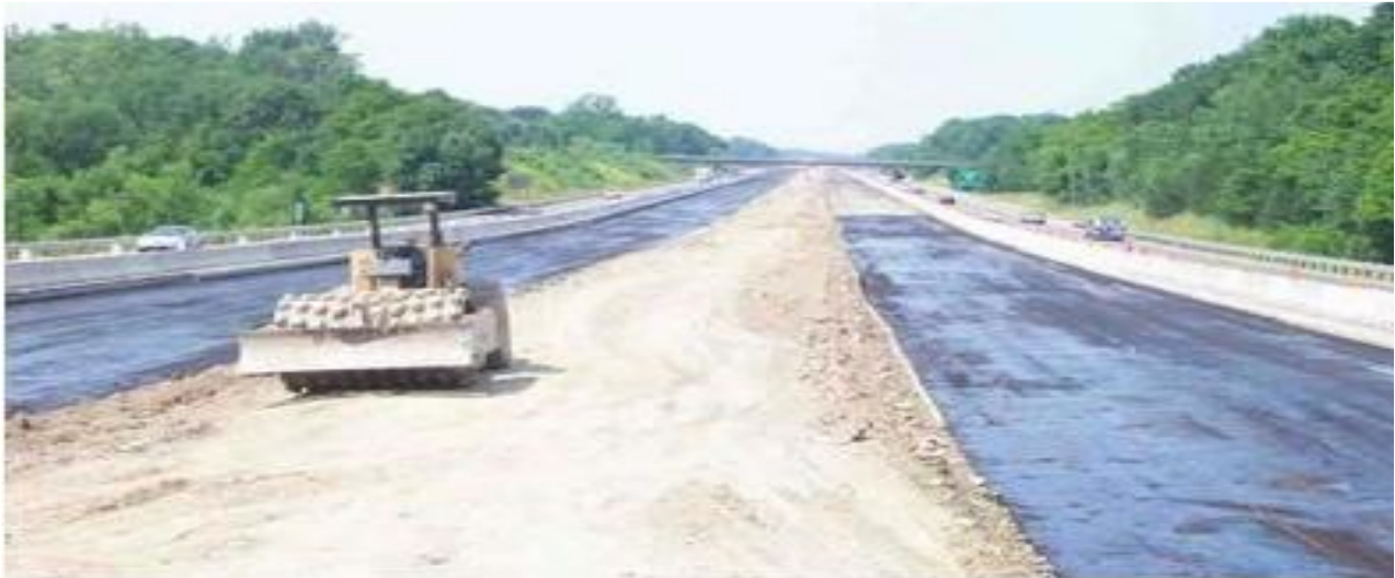
Fig. 7 Prime coat emulsion for curing
