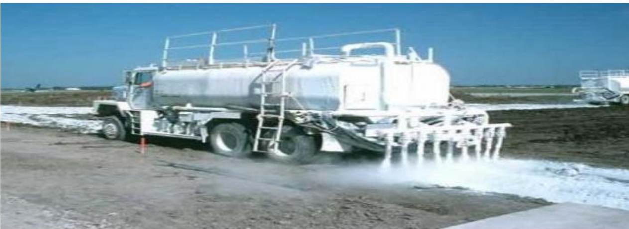
Fig. 3 Spreading of lime over scarified soil
