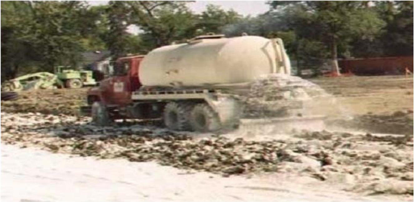
Fig.4 Adding water after dry lime application
