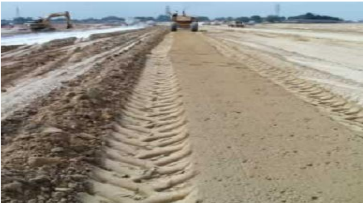
Fig. 5 Mixing and pulverization
