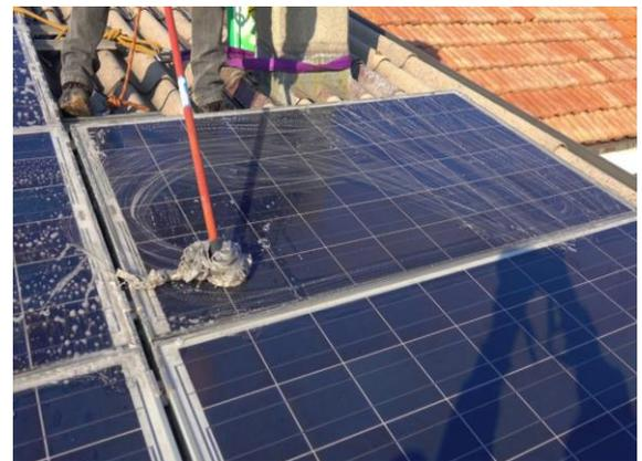
**Fig.2: Manual Cleaning of Solar Panel**
