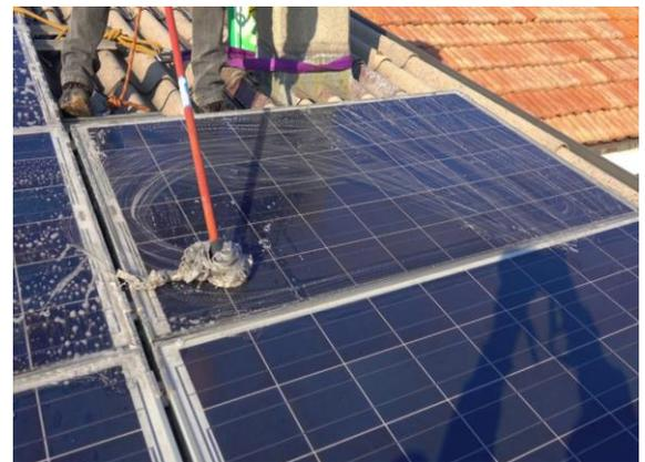
**Fig.2:Manual Cleaning of Solar Panel**
